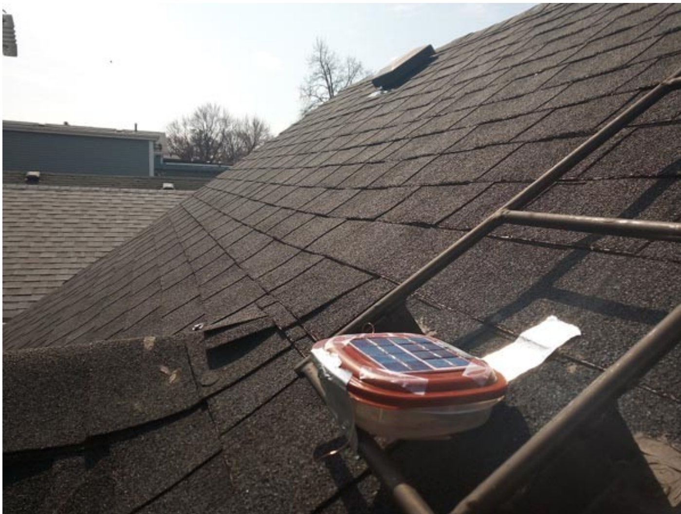
Using a food container to do solar roof testing of a U4B
